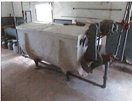
The bases of many pieces of equipment and furnishings are embedded in the concrete floor, sometimes encased in metal forms that have seriously corroded due to periodic flooding.
