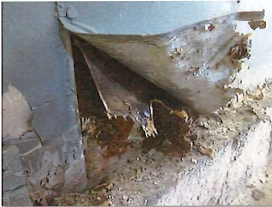
This exposed exterior sill plate shows evidence of rot.
