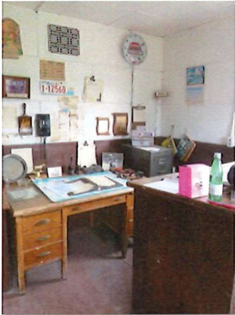
The floor in the office is plywood.
