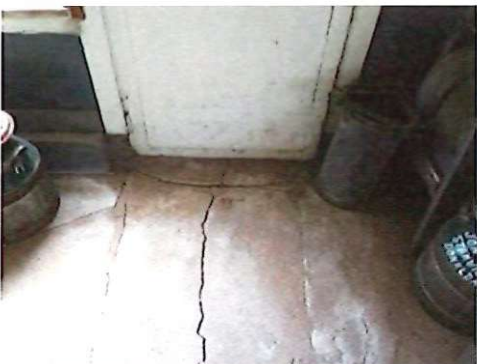
These images illustrate the poor condition of the concrete floor slab.
