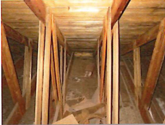
The fabricated roof trusses over the main portion of the Creamery
