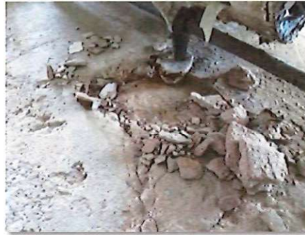
The concrete topping is flaking off in places.
