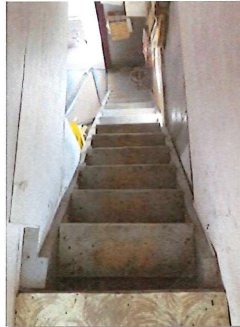
The stairs to the attic office are wood.
