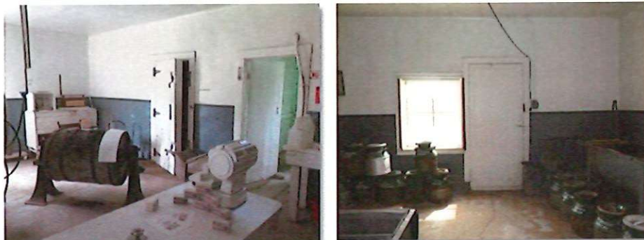
Painted metal-clad walls and ceiling in the pasteurization room
