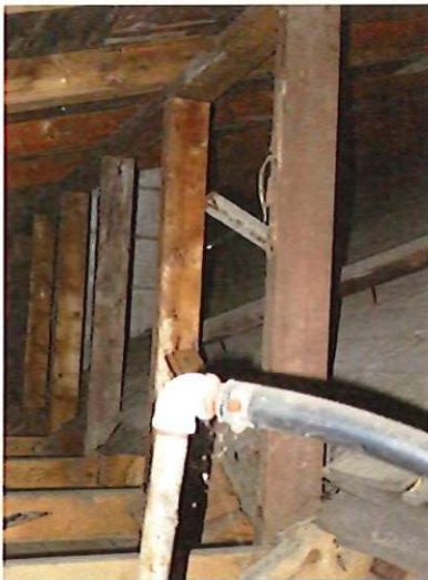
The original machine shop roofing is under the roof of the east addition
