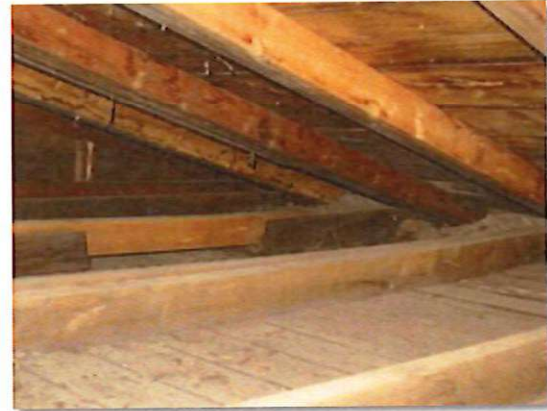
The 2x4 roof joists over the east addition
