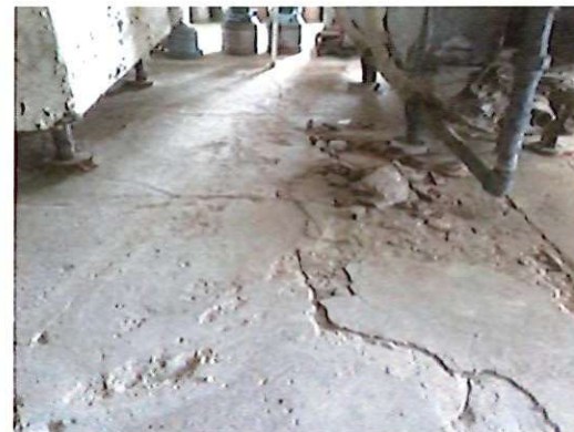
The bases of many pieces of equipment and furnishings are embedded in the concrete floor, sometimes encased in metal forms that have seriously corroded due to periodic flooding.
