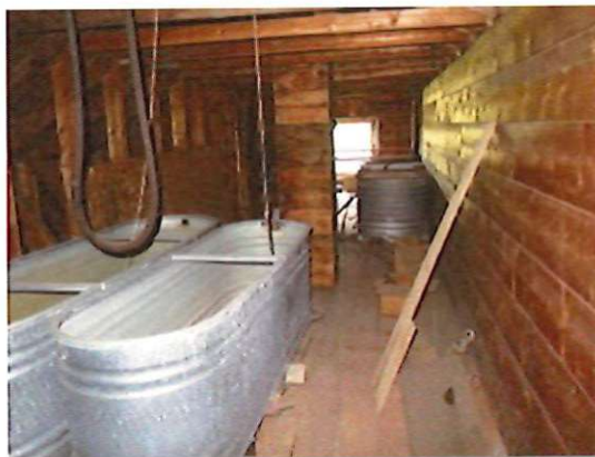
The attic 'room' inserted into the trusses
