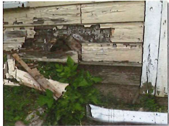
The base of the rear wall has been exposed to moisture.
