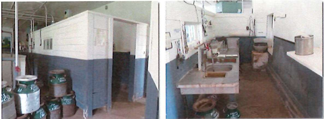
The laboratory testing room partition is constructed from wood boards, which are in good condition.
