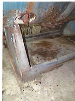
The outer casing of the boiler has severely rusted, exposing the insulating material (asbestos-containing).
