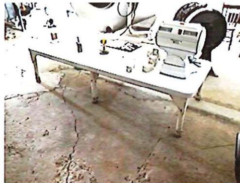
These images illustrate the poor condition of the concrete floor slab.
