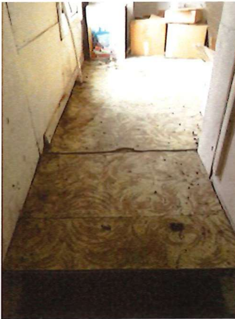
The floor in the attic office is sheet material.
