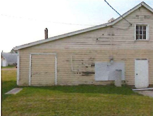
The electrical meter is located on the rear elevation.
