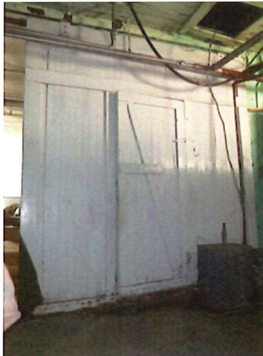
The sliding wood door in the boiler room
