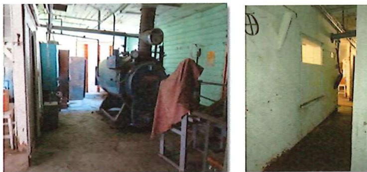
Painted wood shiplap in the boiler room
