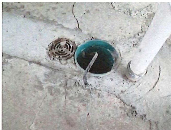
The new floor drain
