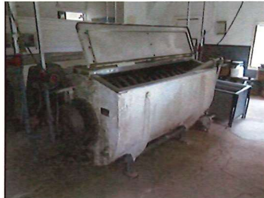
The pasteurizers need to be repainted.
