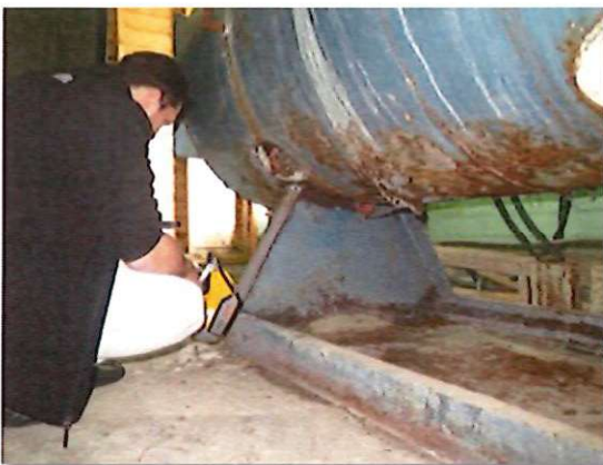
The outer casing of the boiler has severely rusted, exposing the insulating material (asbestos-containing).
