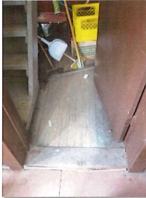
The floor in the attic access room is hardwood.
