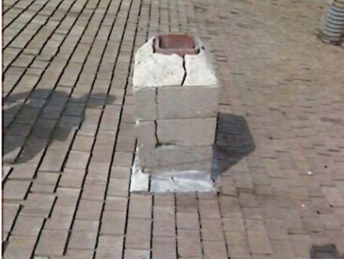
The exterior of the masonry chimney is cracked
