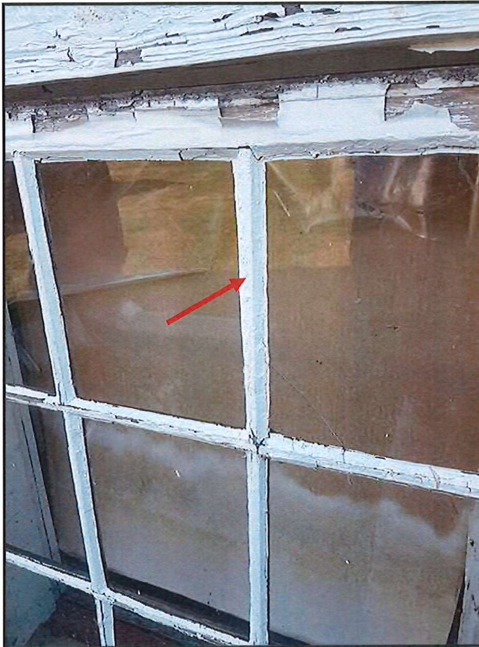
FIGURE 9: WHITE LEAD-BASED PAINT ON WOOD WINDOW MUNTIN, NORTH SIDE OF BUILDING EXTERIOR
